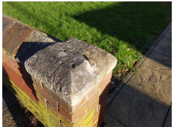
Above: 194 Park Road. This large building, which is now turned over to flats, has a long, low wall. In this instance the railings were cut off with an oxy-acetylene torch. The cut-off 'stubs' can still be seen all along the wall, embedded in their old lead fixings.
