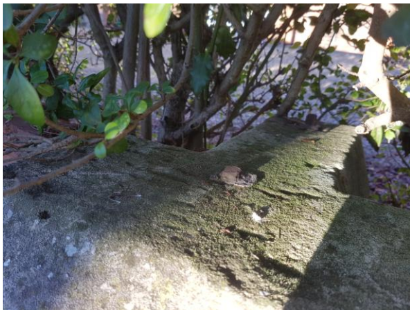
Above: 195, Park Road. Another large building with a low wall from which the railings have been cut using a hot torch.
