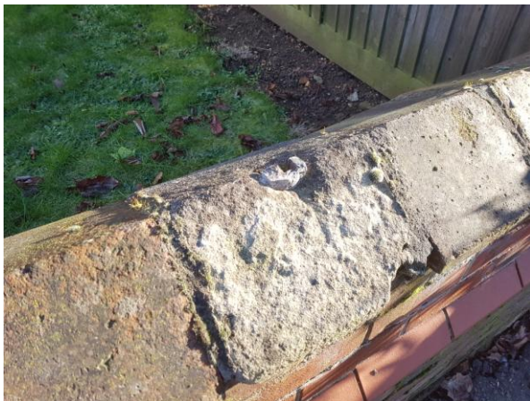
Above: 194 Park Road. This large building, which is now turned over to flats, has a long, low wall. In this instance the railings were cut off with an oxy-acetylene torch. The cut-off 'stubs' can still be seen all along the wall, embedded in their old lead fixings.
